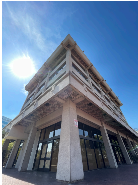
Figure 2: Building corner and roofing underside, JACCC, Los Angeles, 2023
